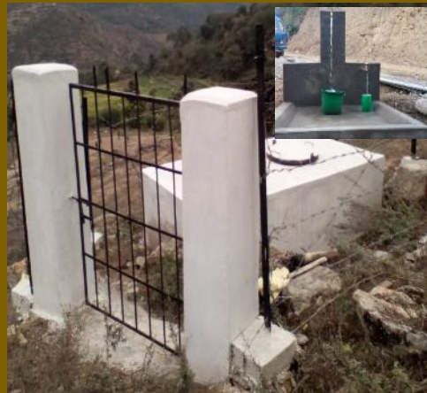
Figure-2 Ghattekhola DWSC – Constructed DC at Bhageshwor RM, 5 Bursa
