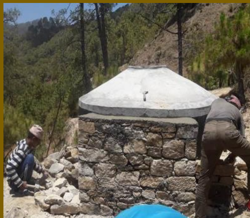
Figure-1 Water Tank Construction at Asurpa DWSP Nawadurga 1
